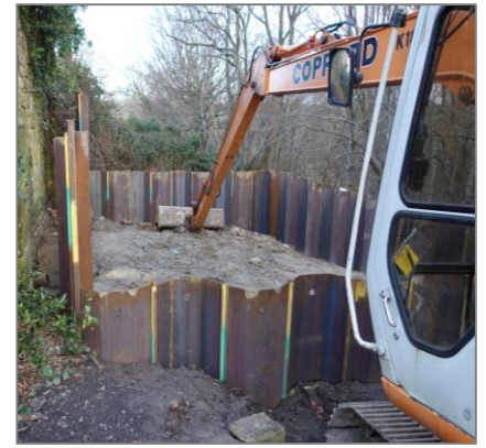
The fuel store being constructed
