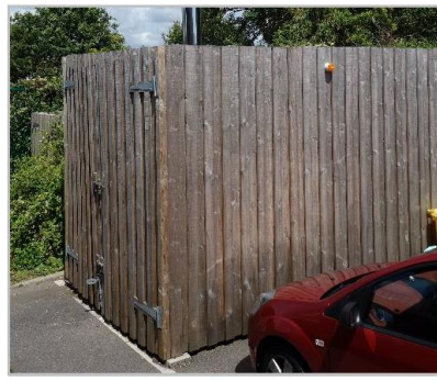
Container, housing the new biomass system
