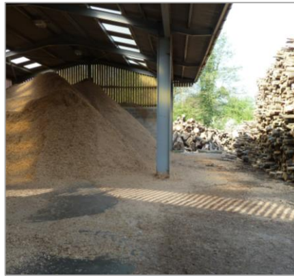
Storage building housing the wood chip, sourced locally
