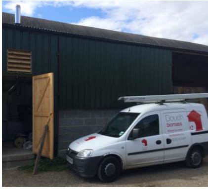
The plant room and fuel storage barn
